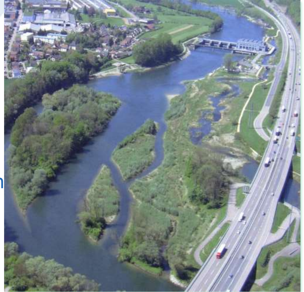
Ruppoldingen run-of-river powerplant, Switzerland
